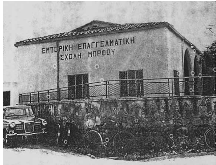
The building of the Morphou School of Commerce.
