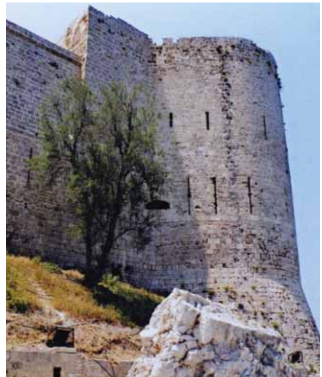
The Lusignan tower on the north-east side of the castle. Photo: Kyrenia Municipality Archive
