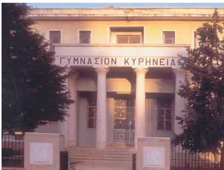
Entrance of the high school of Kyrenia.
