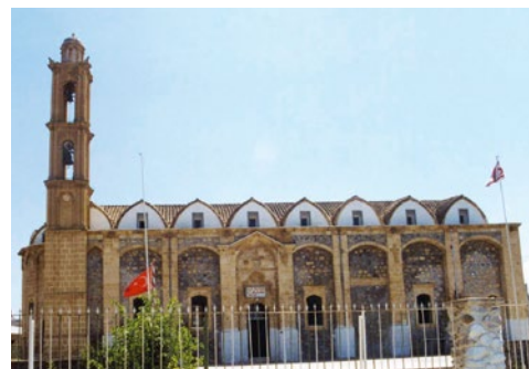
381. Church of Timios Stavros , KATO ZODEIA (Converted into Mosque)
